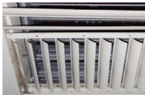
AFTER CLEANING BY COIT
